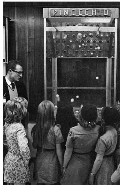
Figure 7. Pinocchio was a “puppet” reactor that used ping-pong balls to simulate nuclear fission, photographed here at the LASL museum in 1966. It demonstrates the types of trajectories that Ulam and von Neumann sought to simulate using the Monte Carlo method. Also known as the popcorn machine, Pinocchio was a star exhibit at the museum. It has recently been reengineered—you can see Pinocchio 2.0 at the Bradbury Museum, along with a forthcoming exhibit on the Monte Carlo method due in 2024.
